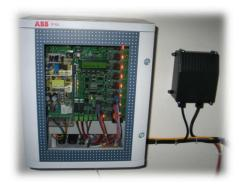
and unlock doors when there is a mains power outage, preventing a "lock in" situation. There should be no reason for the owner to enter this control box.
